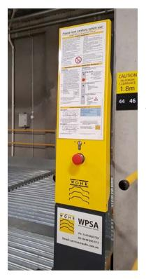
The users operate the system via an easy to use key switch, which is hold-to-run for the safety of vehicles and pedestrians in the area.
